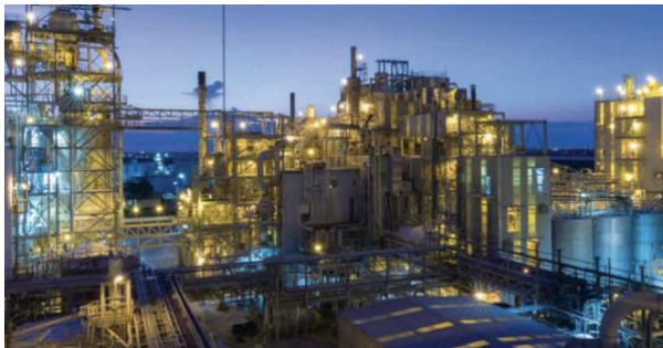
An Albemarle bromine manufacturing plant
